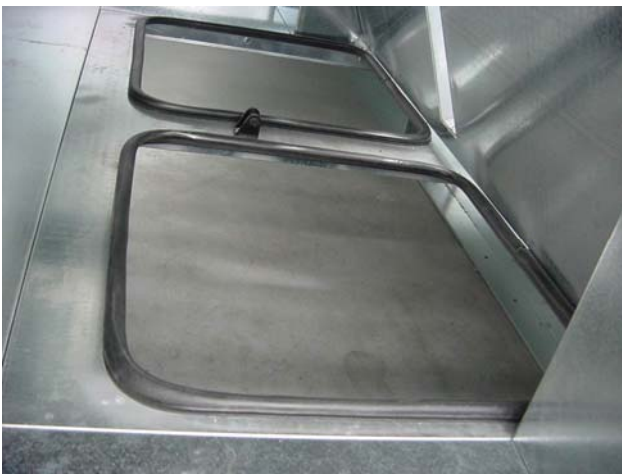
POSITION OF THE SEALS ON THE RECIRCULATION DAMPERS
