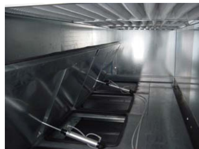
BYPASS DAMPER OPEN ( BAKING OR RECIRCULATION PHASE )
